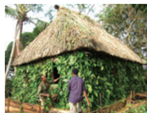
Reconstruction project of Fijian traditional wooden house “Bure”
