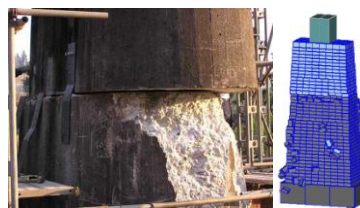
Fig.1 Horizontal gap on the cold joint 2) (left) and Reproducible analysis(right)
