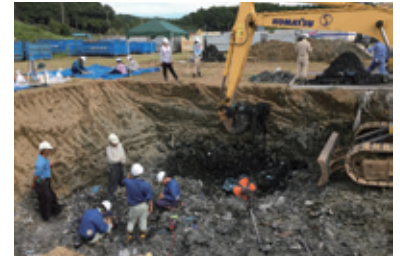
Site investigation at a waste landfill site
