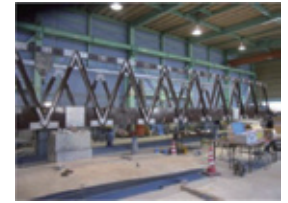
Durable FRP Bridges
