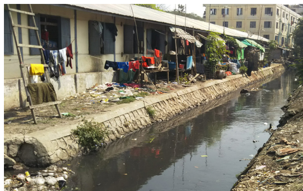
An Open Drain in a Residential Area of Mandalay, Myanmar
