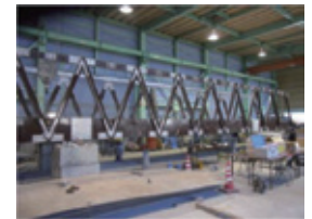
Durable FRP Bridges
